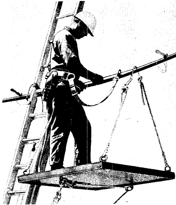
Fig. 8—Method of Using Safety Strap When Working From Aerial Platform
